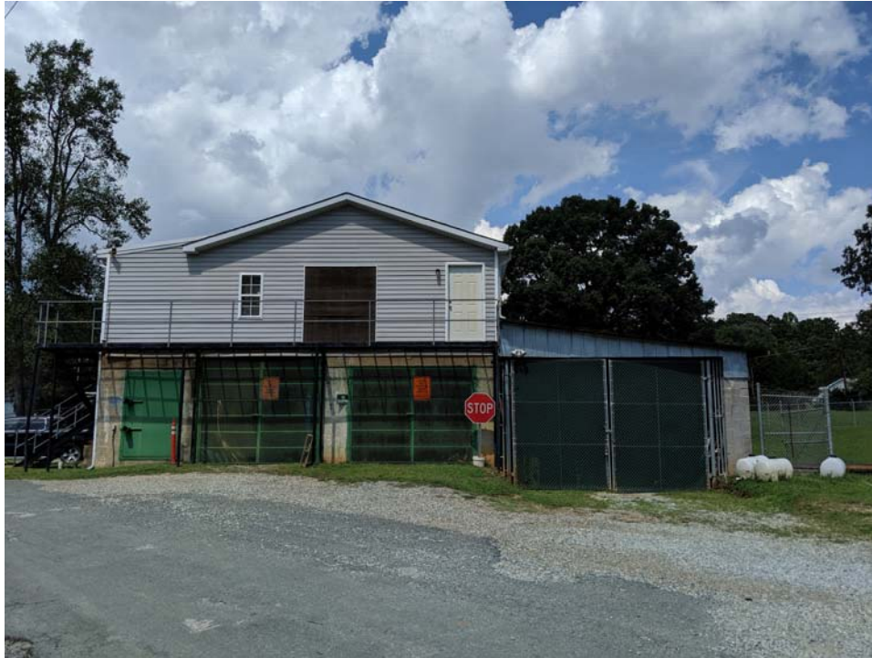
715 Dimmocks Mill Road Water Plant C Side
