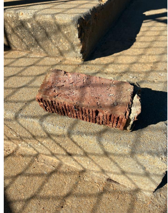
Figure 3 – Sample of Existing Brick located On-Site to repair NE Foundation
