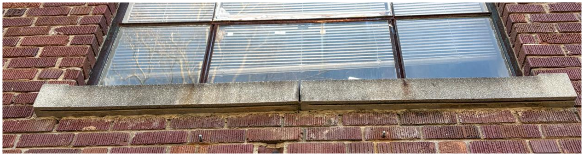
Figure 1- Existing 2-Piece Window Sill
