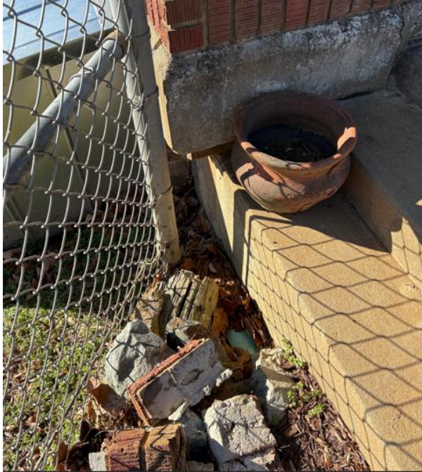
Figure 2 - Existing Brick onsite to repair NE foundation – Foundation corner visible where repair is needed.
