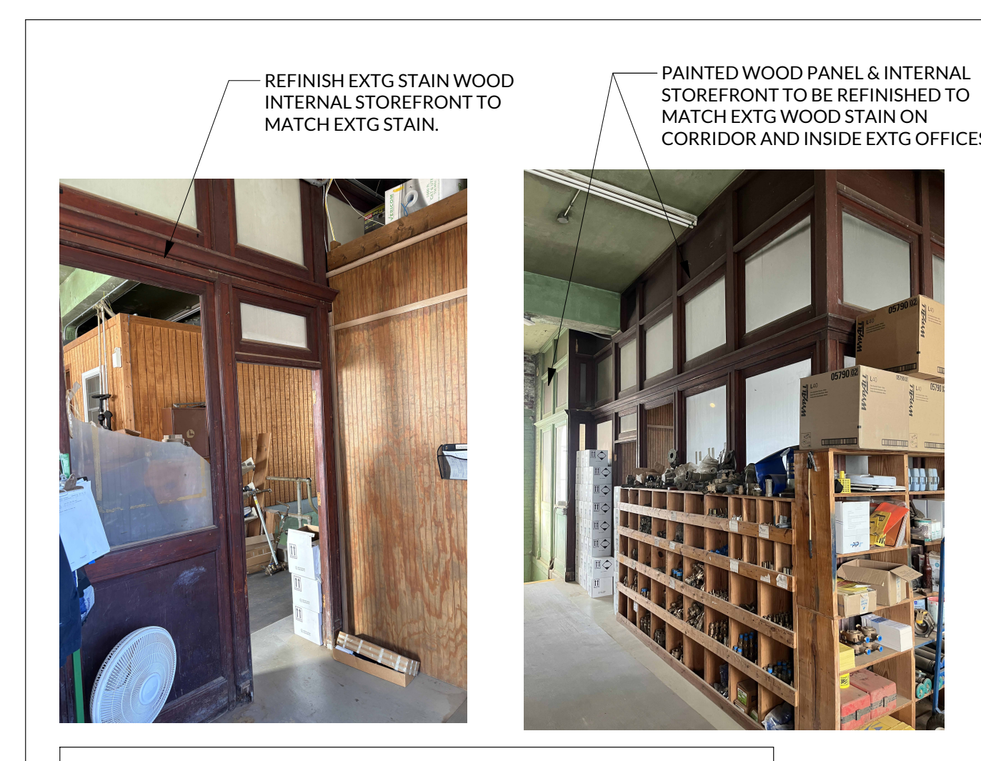
REFERENCE NOTE - T, EXTG INTERIOR WOOD STOREFRONT
